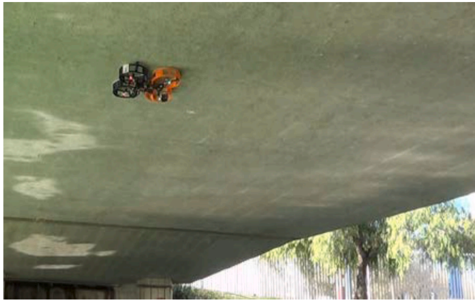
Fig. 9. Drone hovering attached to bridge intrados [114].
